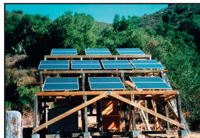
Photo Courtesy of Solar Electric, Inc.
